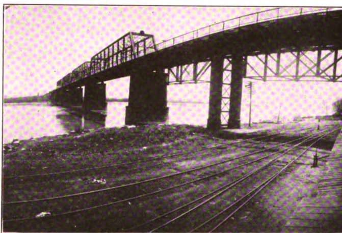
Present Railroad Bridge Across Missouri River
