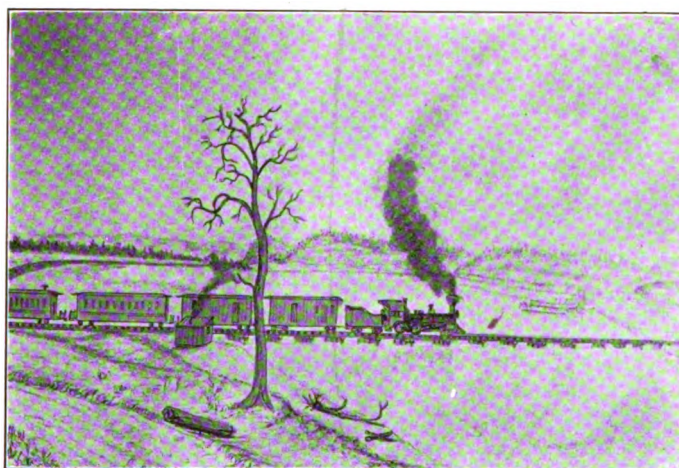
First Temporary Bridge and First Train Crossing the Missouri at Omaha 1866
