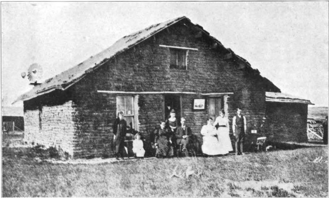
J. C. BERRY AND FAMILY. Typical Sod House Erected in 1891. Sheridan County, Nebraska.
