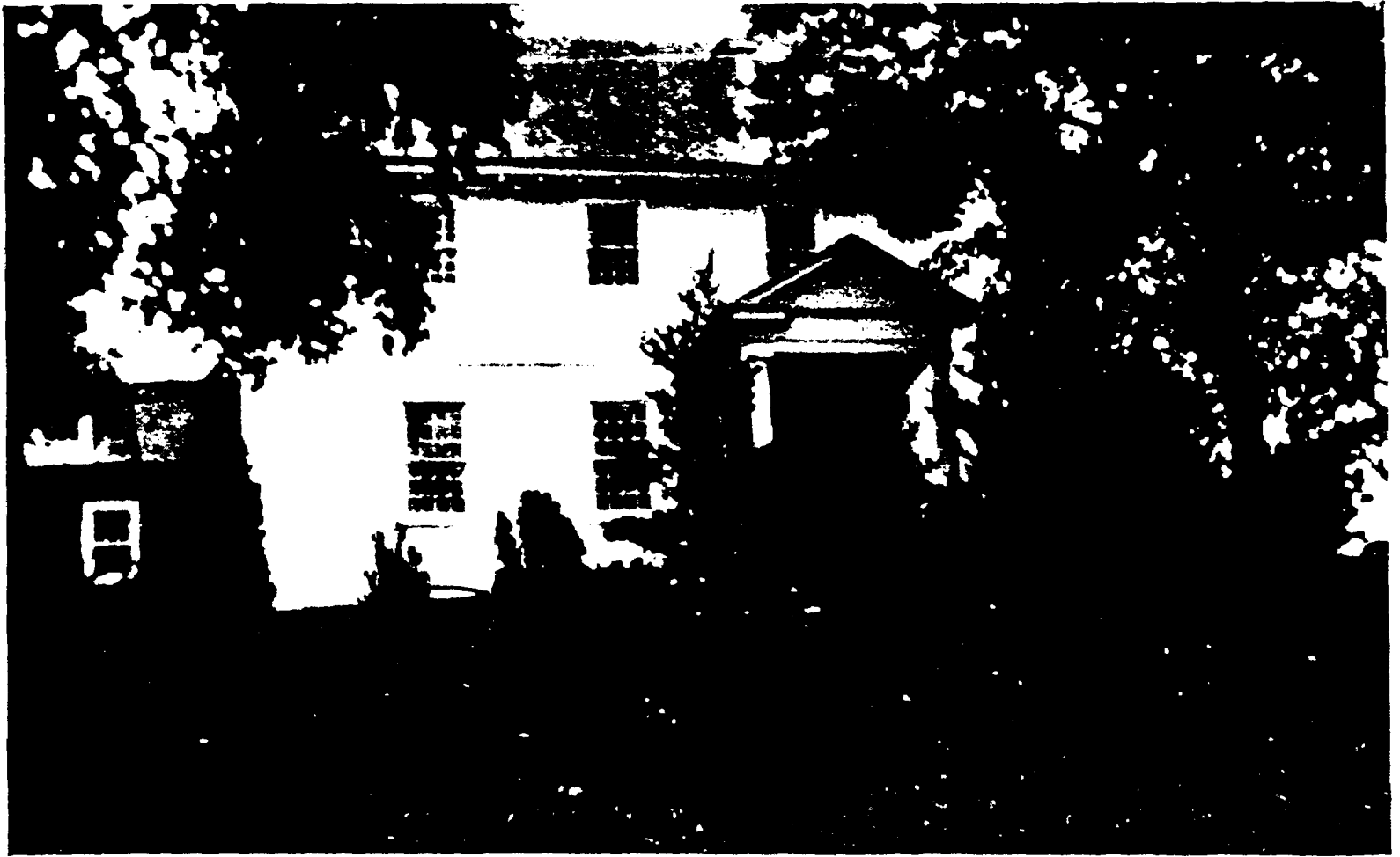
AN UNUSUAL STUDY OF LIBERTY HALL OVERLOOKING THE NANTICOKE RIVER Built by Captain John Smoot of Rehoboth, Dorchester County, Md.
