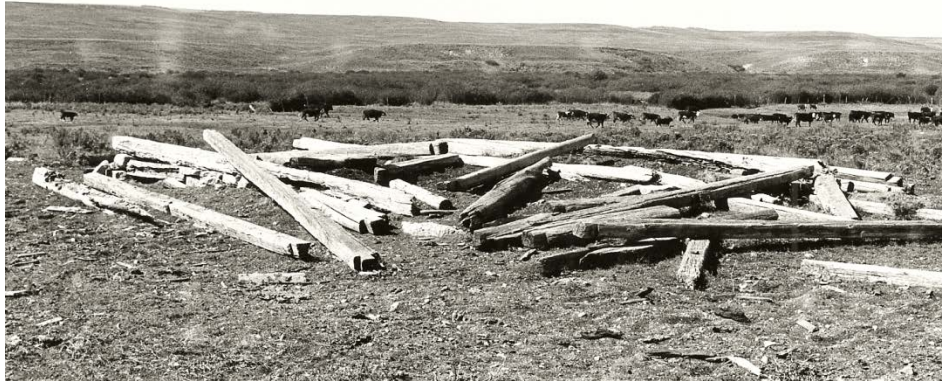
Ham's Fork School (1897) Ruins, Lincoln County (Wyoming Cultural Sites Inventory Form, 1983, State Historic Preservation Office)
