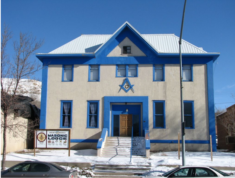
Former Green River elementary school, now a Masonic Lodge (Mary Humstone, 2006)
