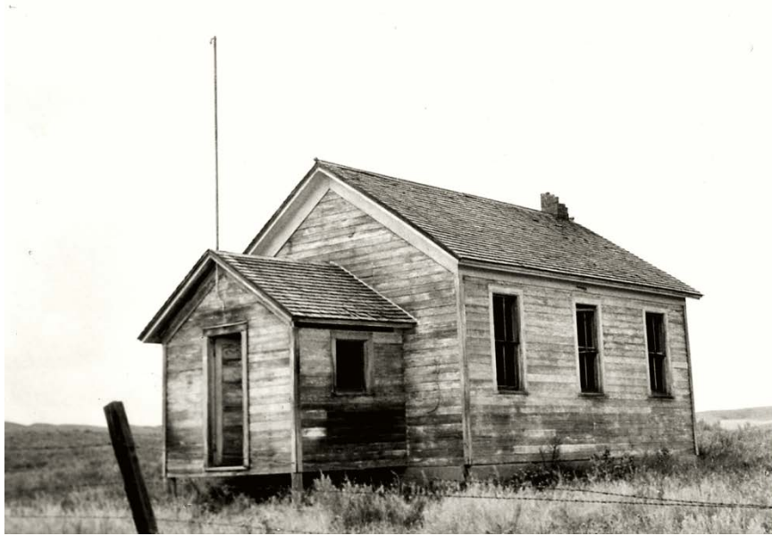
Owen School (Little Blue School), Moved to Ranchester, Sheridan County (Wyoming Cultural Sites Inventory Form, 1981, State Historic Preservation Office)
