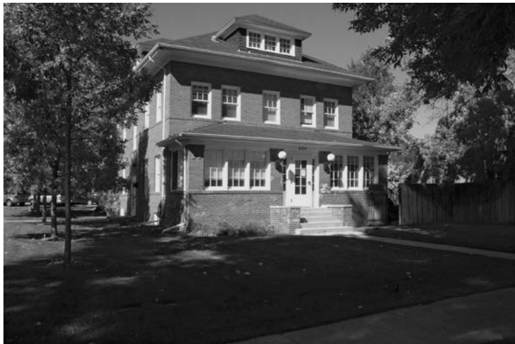
Original School built for the Blind (1887), Cheyenne, Laramie County (Richard Collier, 2009, State Historic Preservation Office)
