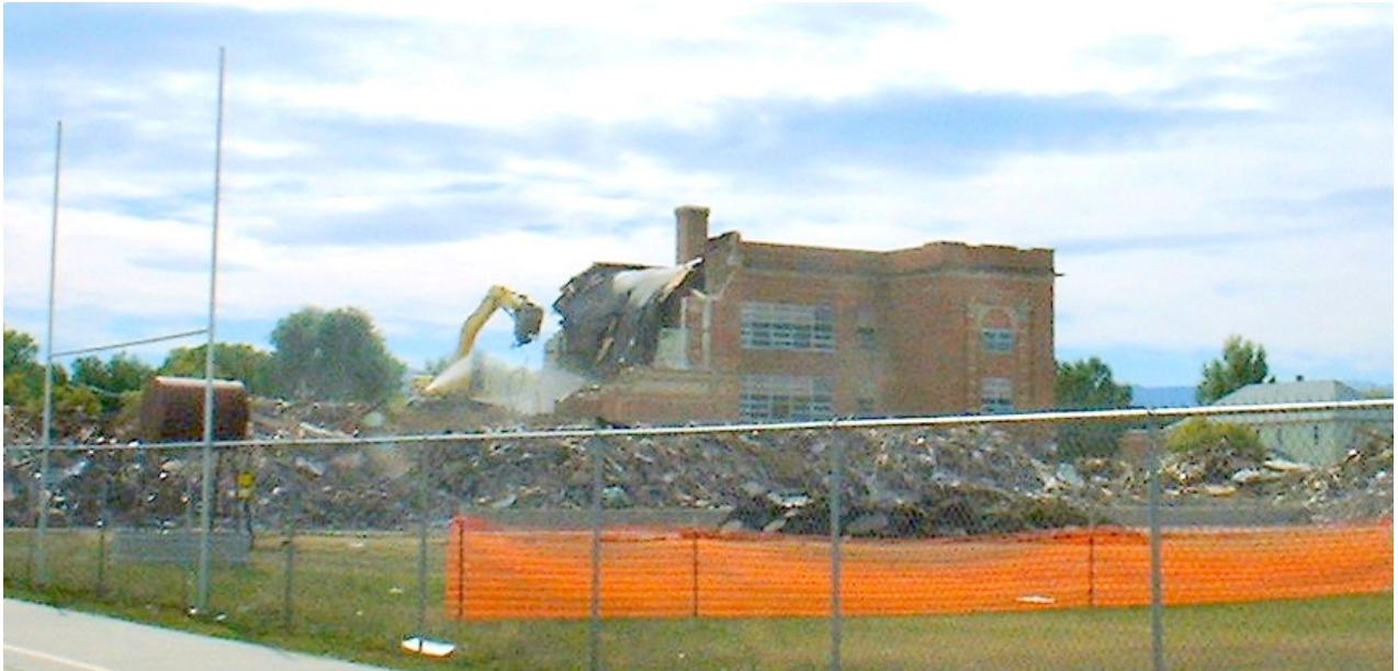
Demolition of Sheridan High School (Mary Humstone)
