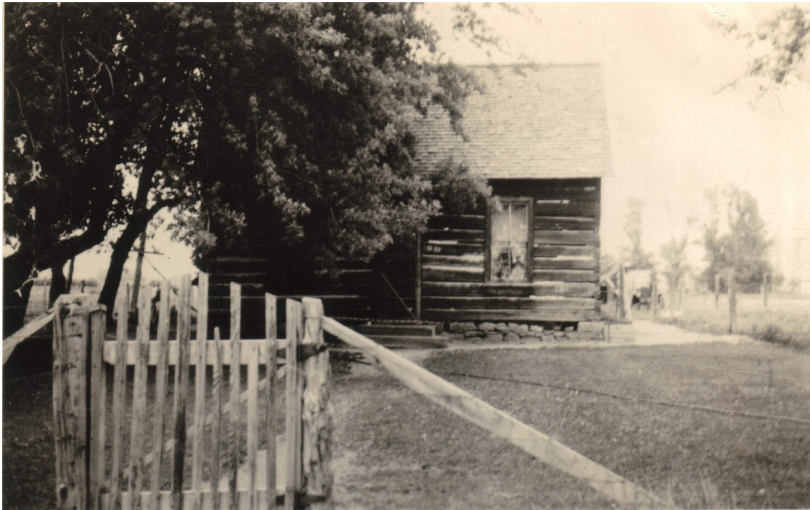
◀◀ Log house at Newton built by Christian Andersen sometime after 1870 and served as their home until his death in 1903. Later it became Black Jack Nelson's place. It remained his home at least through the 1920 census and his leaving Newton. Picture was taken a few years after Jack left Newton and after most of the trees and brush had been removed. Picture courtesy of Larry D. Christiansen.
