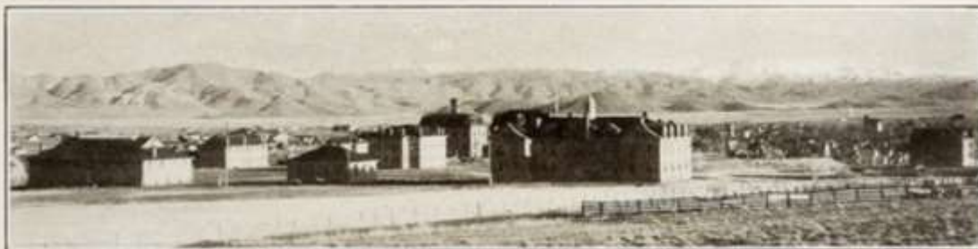
General View from the Northwest
