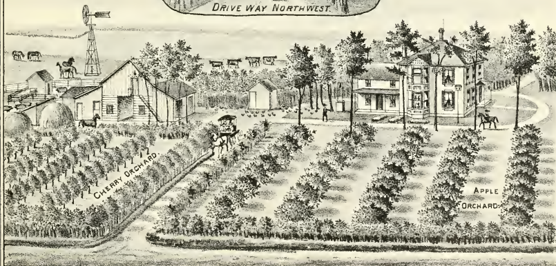
RESIDENCE OF E. O. WAIT, SEC. 9. STEVENS CREEK PRECINCT.
