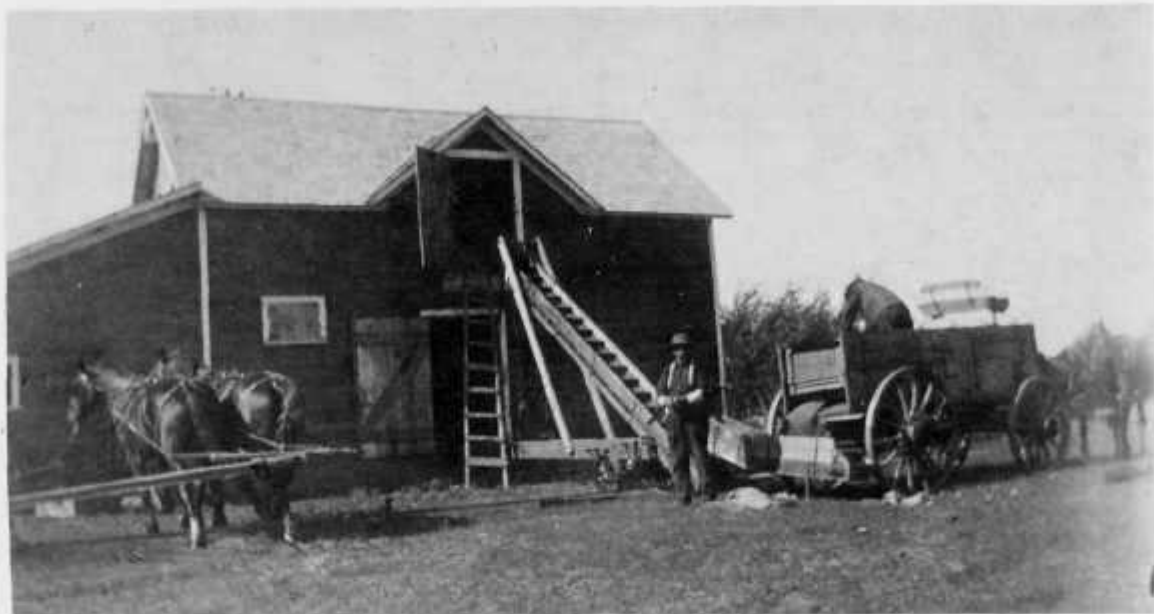
This picture shows the wooden auger used on the John Dutee, Jr. farm in 1914. The horses went in a continuous circle to provide the power. The horses were trained to step over the rod as they made their circle.
