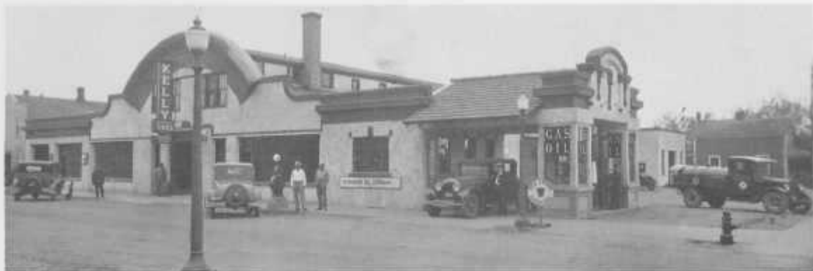
The Carson Garage in what was recently the Archie Campbell building and today is occupied by Topp's Feed & Seed.
