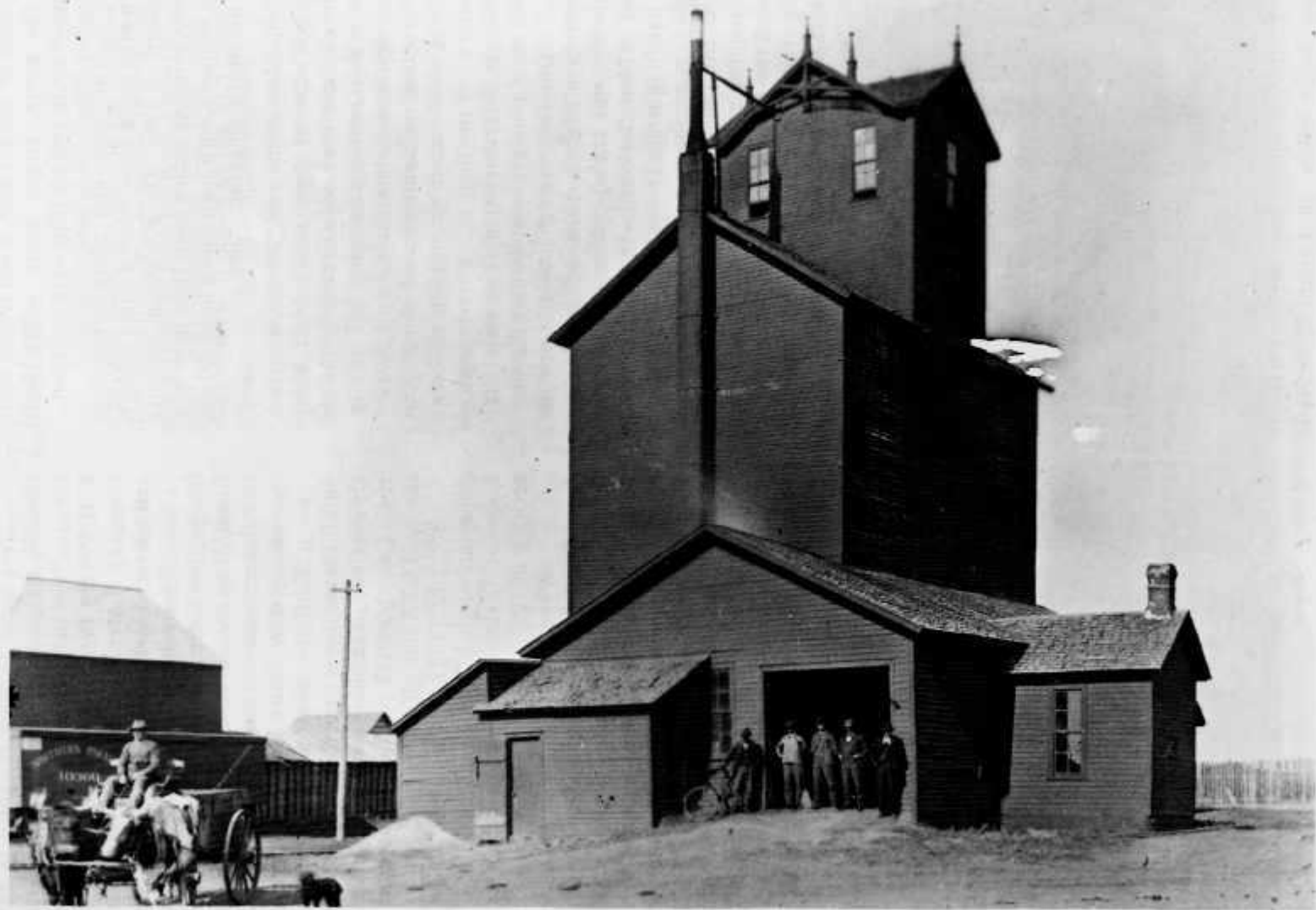
This structure is thought to be the Monarch-Peavey Elevator at New Rockford
