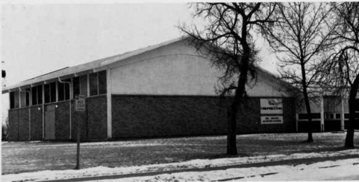
Westside Elementary School here has been abandoned as enrollment dwindles and the structure converted into a Tri-County Activity and Learning Center for the developmentally disabled citizens of the state.
