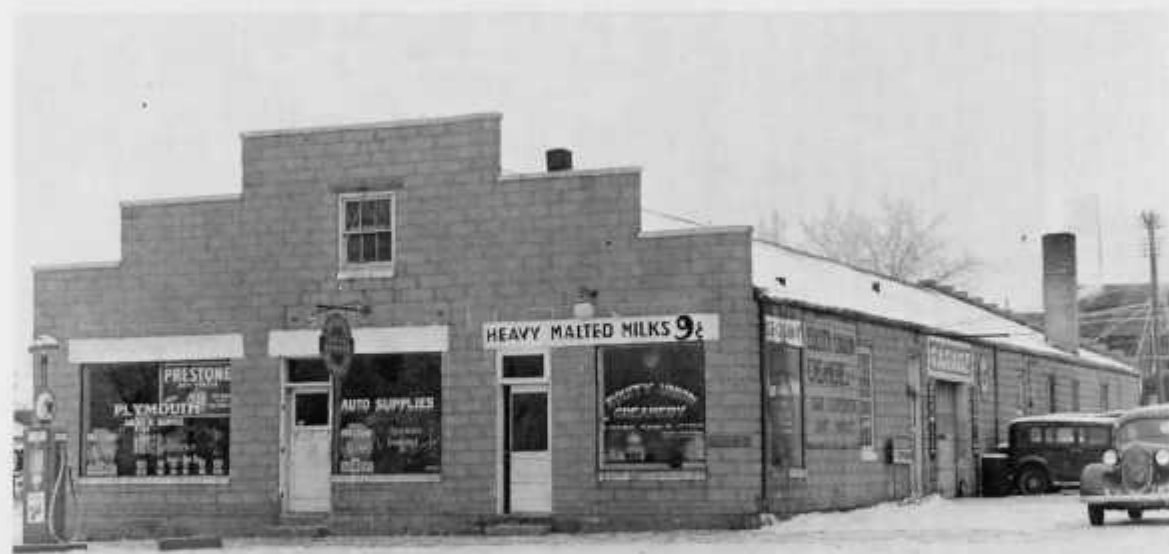
Foster's Garage and Auto Supplies (now Foster's GTC Auto Parts) is shown in this photo believed to have been taken in the 1930s. The building is thought to have been constructed with Culp's handmade cement blocks. —Photo contributed by Ivon Foster
