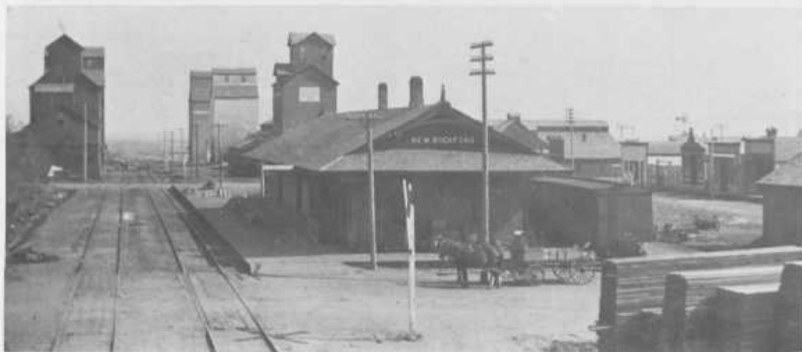
Typical New Rockford Elevator Scene
