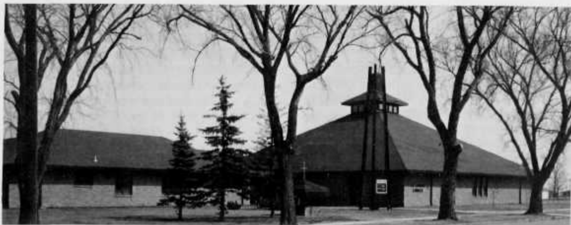
The present St. Johns Catholic Church built on the site of the old St. James Academy. Ground was broken May 13, 1977, and the complex was dedicated June 18, 1978.
