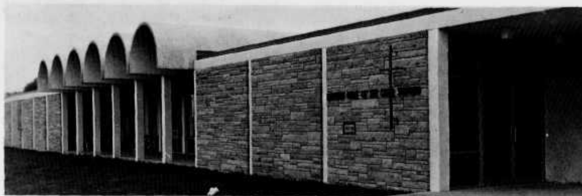
Lutheran Home of the Good Shepherd showing the entrance area and an alcove where residents can sit just off the dining area.
