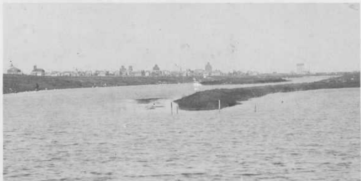
Looking toward New Rockford from the northeast, the date of this photo is not known. The flour mill is barely visible at right, and a smokestack issuing a plume of smoke in the center is thought to be New Rockford's Municipal Power Plant.
