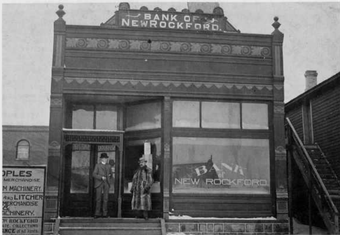
The Bank of New Rockford was organized in 1881, two years before New Rockford was established as a city. It was located in a building near the spot now occupied by Joe's Knotty Pine. It later moved to the building now occupied by the American Legion. Pictured on the steps of the bank are Mr. Severson and W. C. Dresser.
