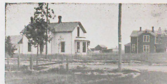
RESIDENCES OF ROBERT S. CRAIG AND FRANK C. DAVIES, NEW ROCKFORD, N. D.
