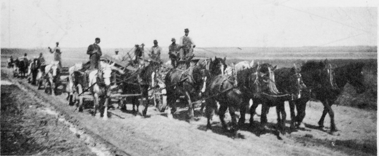
Typical road building scene.
