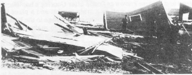
Results of tornado at Westhope, 1909.
