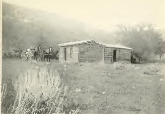
THE "HOLE-IN-THE-WALL" CABIN
