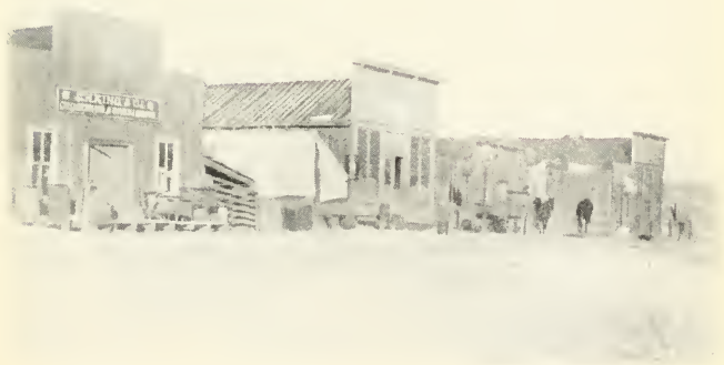
NORTH SIDE OF MAIN STREET IN 1888—"OLD TOWN" OF CASPER
