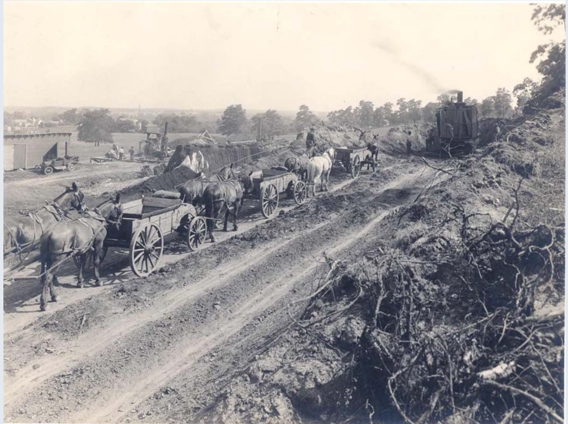
Possibly Jefferson St construction during excavation for Handley High School- June 1921
