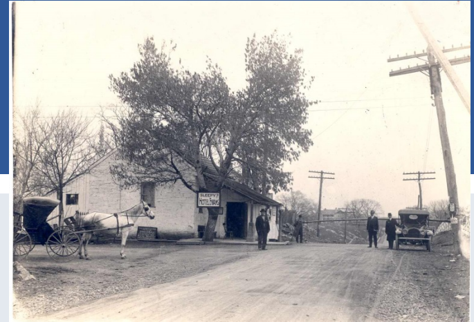
Hillman Toll- Valley Pike at Cedar Creek Grade
