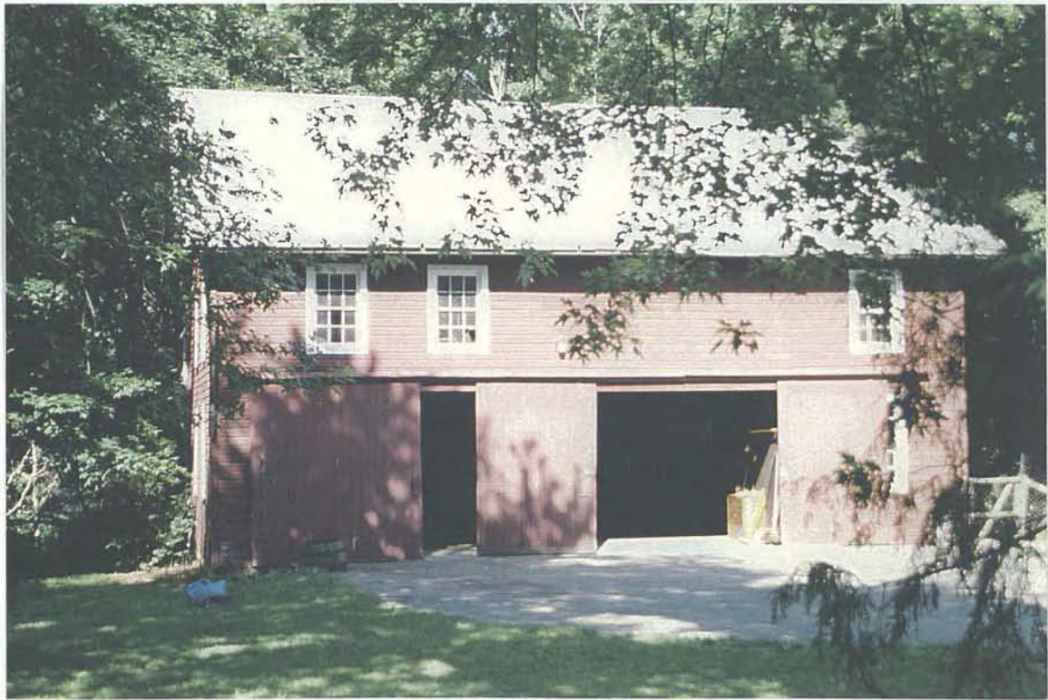
Photographs of Bryan House Additions and Barn
