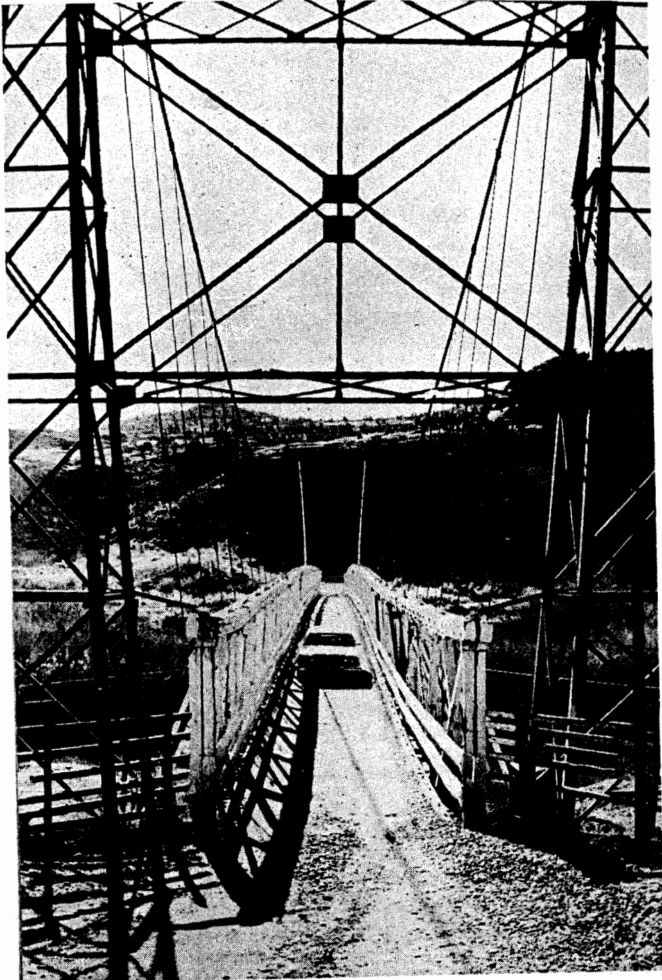
The Dewey Bridge today retains much of its old character.
