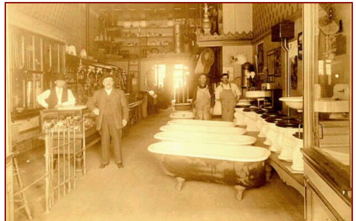
Inside view (early 1900's) of Chris Waltz when located in the 300 block of Woodard. Left to right: Hugo Koeppen, office manager Christian Waltz, owner; Mr. Katchel, Mr. Heimberger
